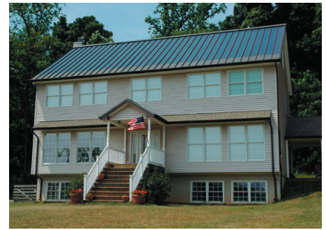
This home on the tour features 36 PVL laminate panels from UniSolar
