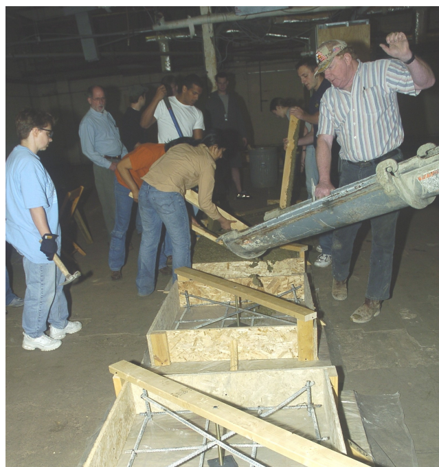
Reds House of ACI/MD Member S&G Concrete Directs the Placing of Concrete in the Footing Forms While Some of the Solar House Students Consolidate and Screed the Concrete
